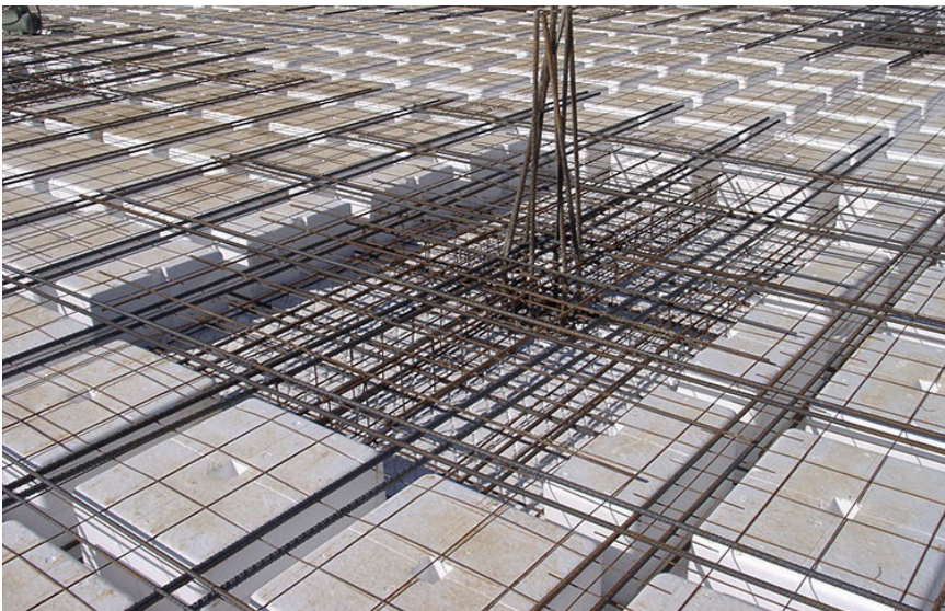
Example of a reinforced concrete lattice slab
