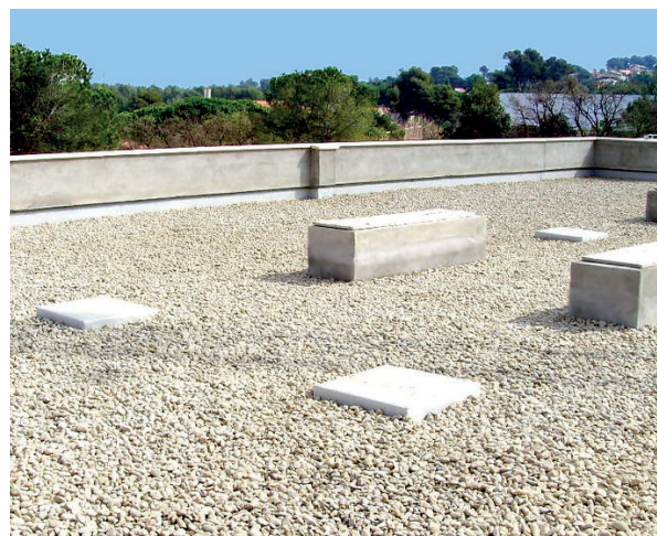
Example of a flat gravel roof
